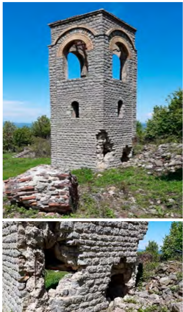
Fig. 2: The bell tower of the Church of Holy Virgin Hodegetria (village of Mushtisht/Mušutište, municipality of Suharekë/Suva Reka) could withstand the attacks by the aggressors in June/July 1999, whose weapons were too “light” to destroy fully the site. Its reinforced concrete construction dates back only to 1989. The 1989 reconstructed monastery could serve its function only for some ten years. The site still lies in ruin, as the Serbian community, which inhabited the place, has meanwhile left and the function of the church has ceased. (photos: author, 5 May 2022)
